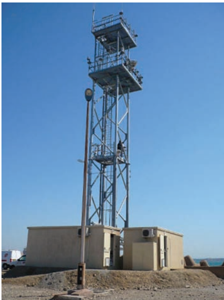
Fig. 2. Pylon and optronic sensors.
